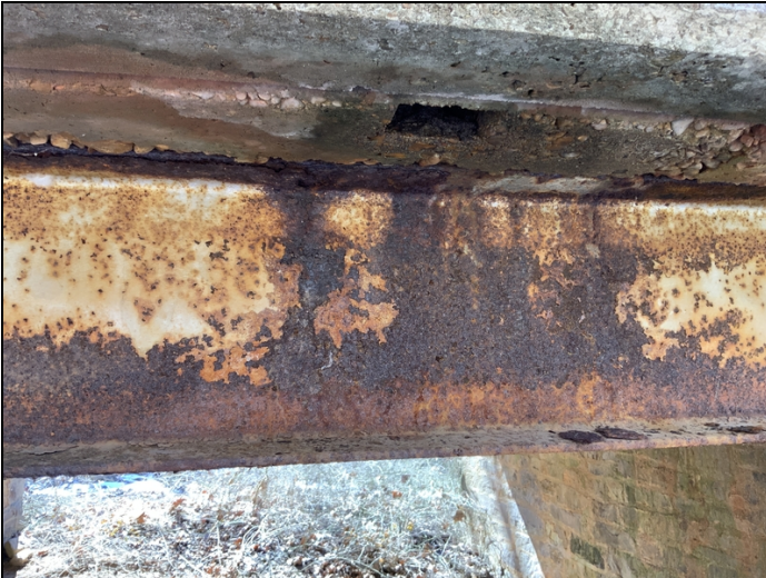
Typ. Rust & Pitting on Outside Beams.
