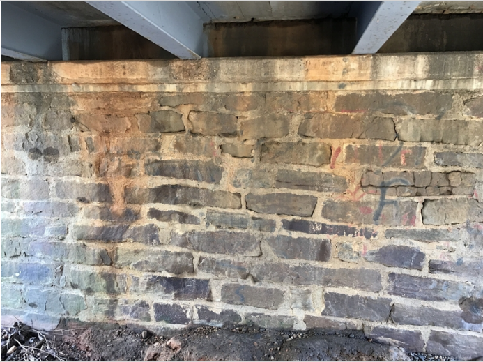
Abutment #5 has minor cracking in a few of the stones and in mortar joints, also there are a few minor spalls in the concrete cap.
