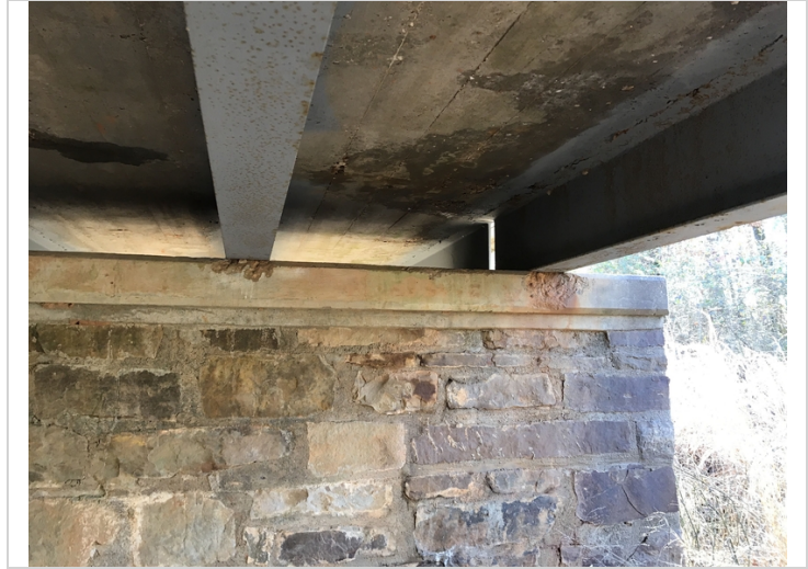
Pier #4 back side has a couple minor spalls under girders 6 and 7.
