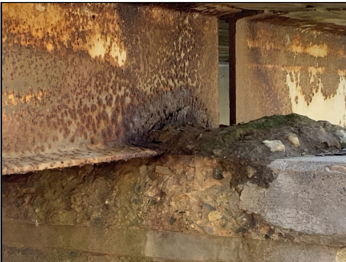
Typ. Rust & Section Loss on Ends of Beams at Piers 2 & 3.
