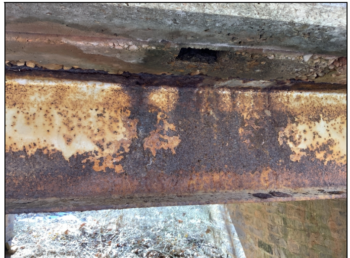
Typ. Rust & Pitting on Outside Beams.
