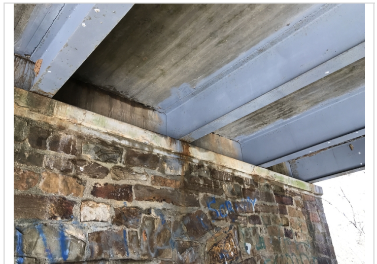
Girders over abutment #1, girders have been painted throughout all spans.
