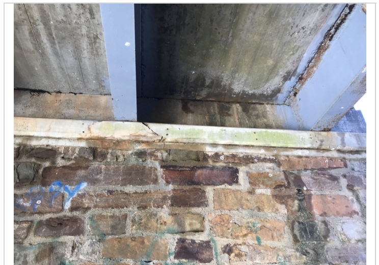
Abutment #1 has some minor delam in the concrete cap under beam #2. There is a couple cracks in the concrete cap.
