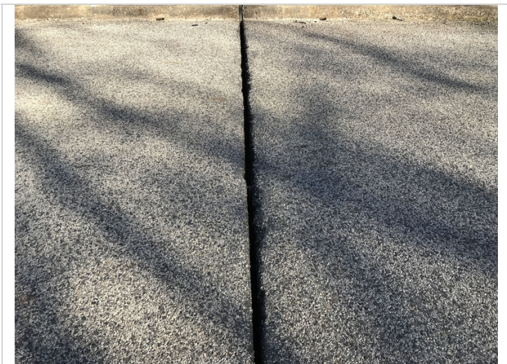
Deck has open joints .
