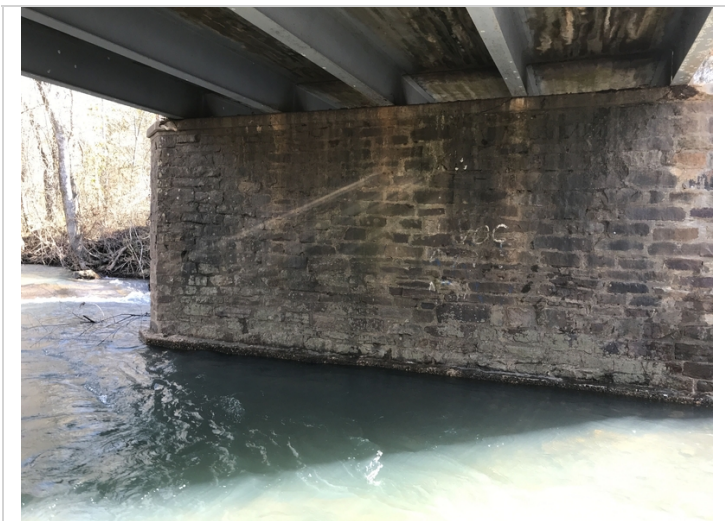
Pier #2 back side has some minor cracking in the mortar joints and some missing mortar in a few areas.
