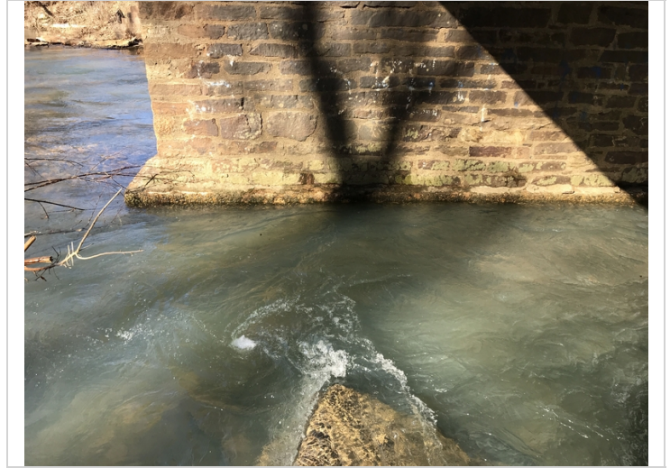
Ahead side of pier #2 has some minor insignificant scour (approximately 18"-24") with no undermining.
