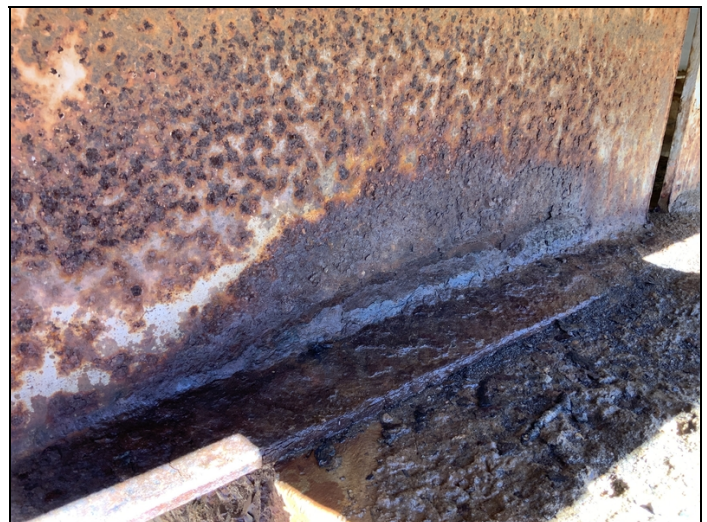
Typ. Section Loss on Ends of Beams.
