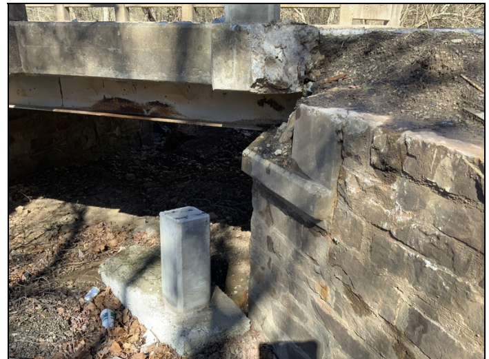
Rail & Curb Broken off at Abutment 5 Rt. Side.
