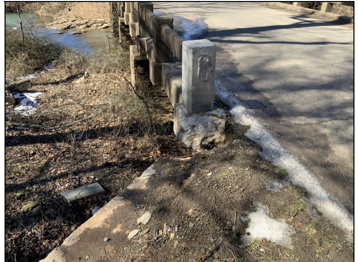
Rail & Curb Broken off at Abutment 5 Rt. Side. East End
