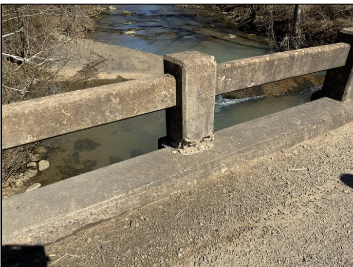
Impact Damage to 1st Rail Post Ahd. of Abutment 1 Lt. Side. West End
