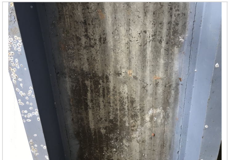
Span #1 has a few minor cracks in the soffit area of bay #4. Typical in a few areas of both spans.
