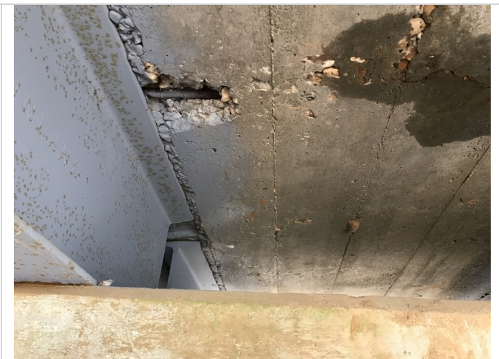
Soffit in bay #5 over pier #4 has minor spall with exposed rebar with no section loss.
