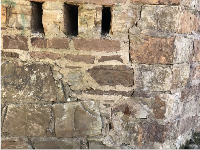
Abutment #1 - Cracking in the mortar joints, few of the stones are cracked in places and mortar is missing in a few areas.
