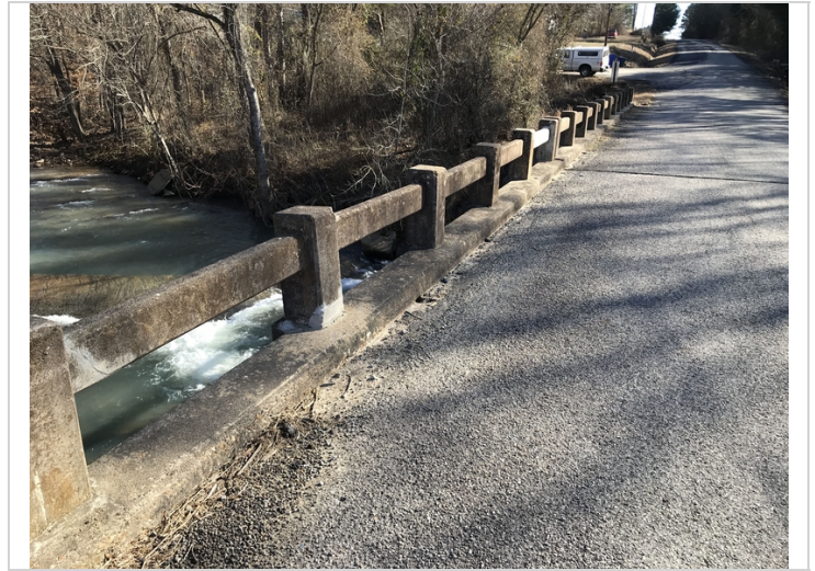
Concrete rail has been repaired and looks good.
