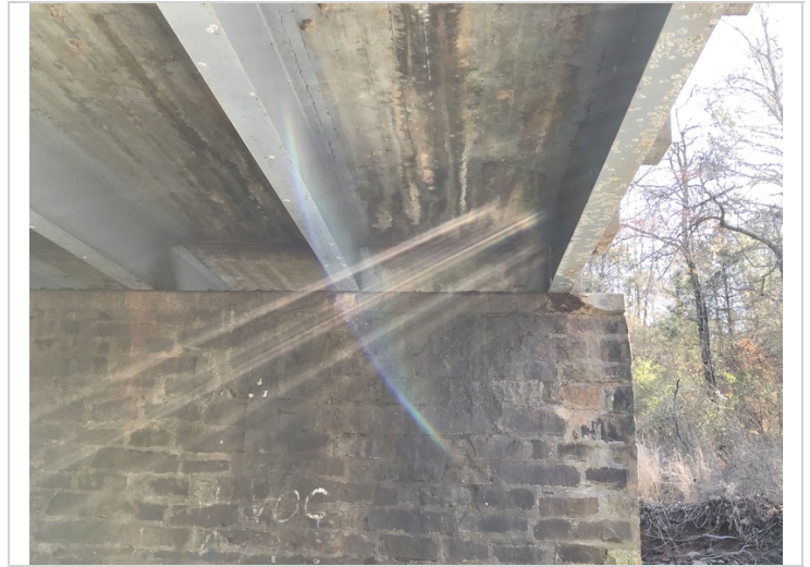
Pier #2 back side has minor spall under girder # 5, there is a moderate crack under girder #4.
