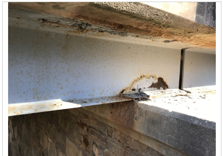
Girder #7 over pier #4 has minor corrosion with minor section loss at the end of the beam. Girder #1 is typical over pier #4.
