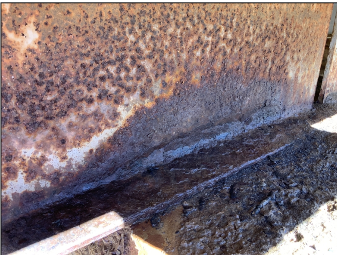
Typ. Section Loss on Ends of Beams.
